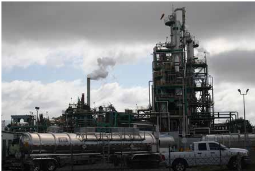
The Evergreen Oil plant in Newark
